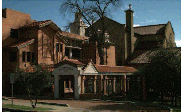
South side of the educational building (formerly the student building).
